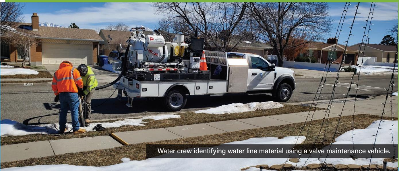
Water crew identifying water line material using a valve maintenance vehicle.
